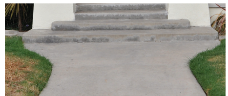
Historic walkways in the Rose Park South Historic District are smooth concrete with scored joints; some "bow" out to meet the edges of the porch steps.
