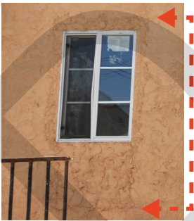
Changing window openings can leave "scars" on the exterior of a building. Red arrows indicate the original extent of the opening.
