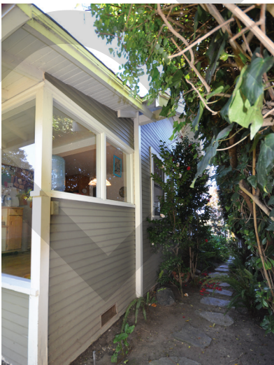
This compatible addition is differentiated from the main house by fixed single-light windows and a vertical strip of wood trim.
