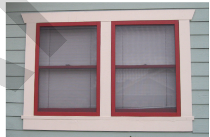
This compatible window screen is sized to the window and has a narrow wood frame painted to match the building's trim.
