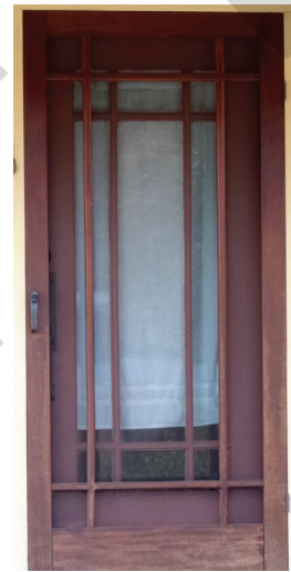
This is an excellent example of a compatible screen door. The narrow wood frame is stained in a neutral color and the mesh enclosure is transparent enough that it does not obscure the door beneath it.
