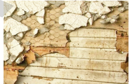
This image shows original wood siding that was incompatibly covered in stucco.
